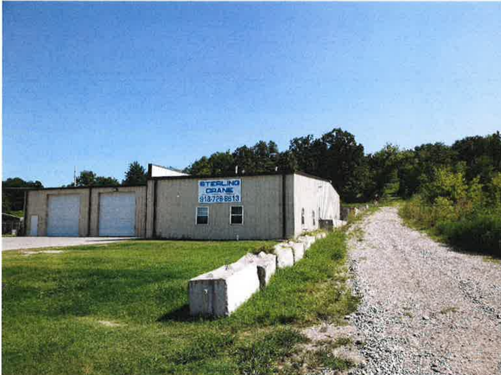
Looking south from W. 21 st St. S. – this driveway appears to go to a house this is also south of the business.
