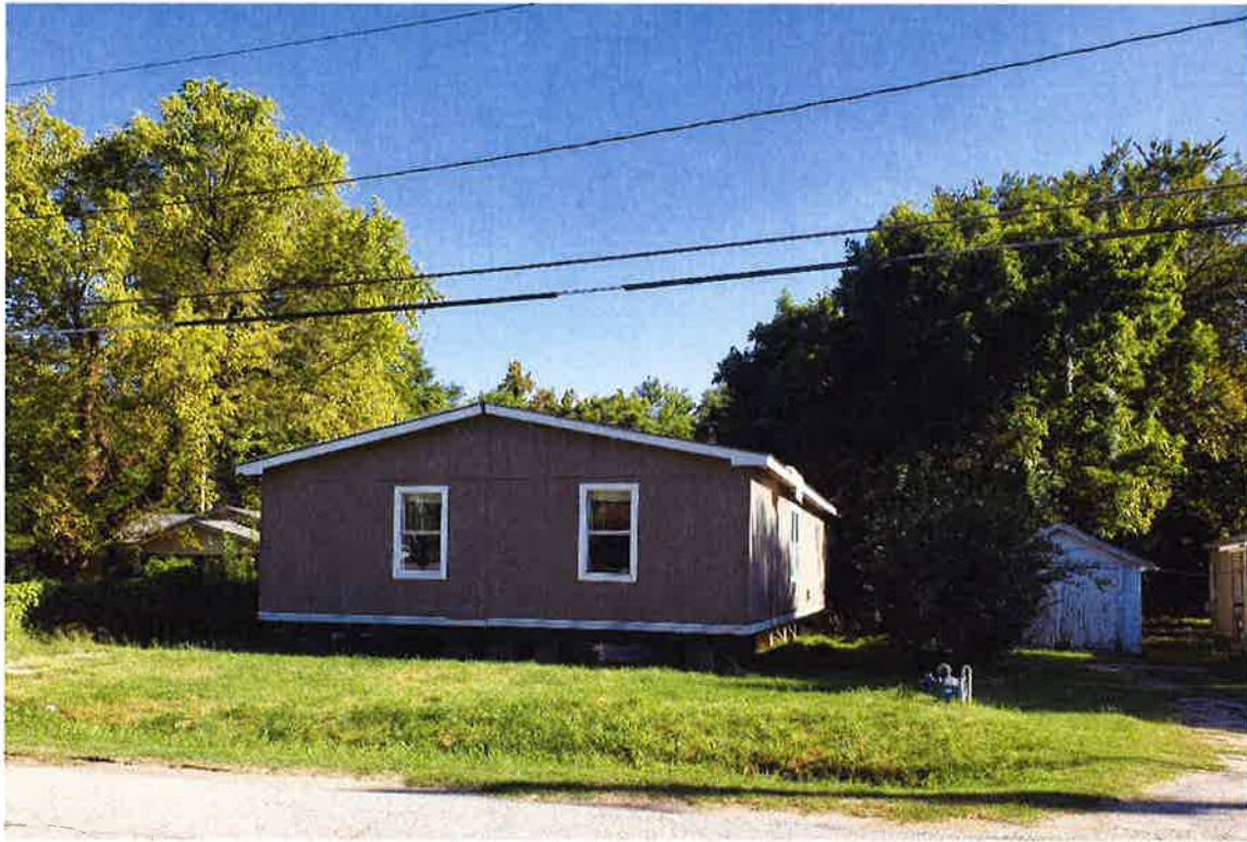
Looking south from W. 4 th St. N.
