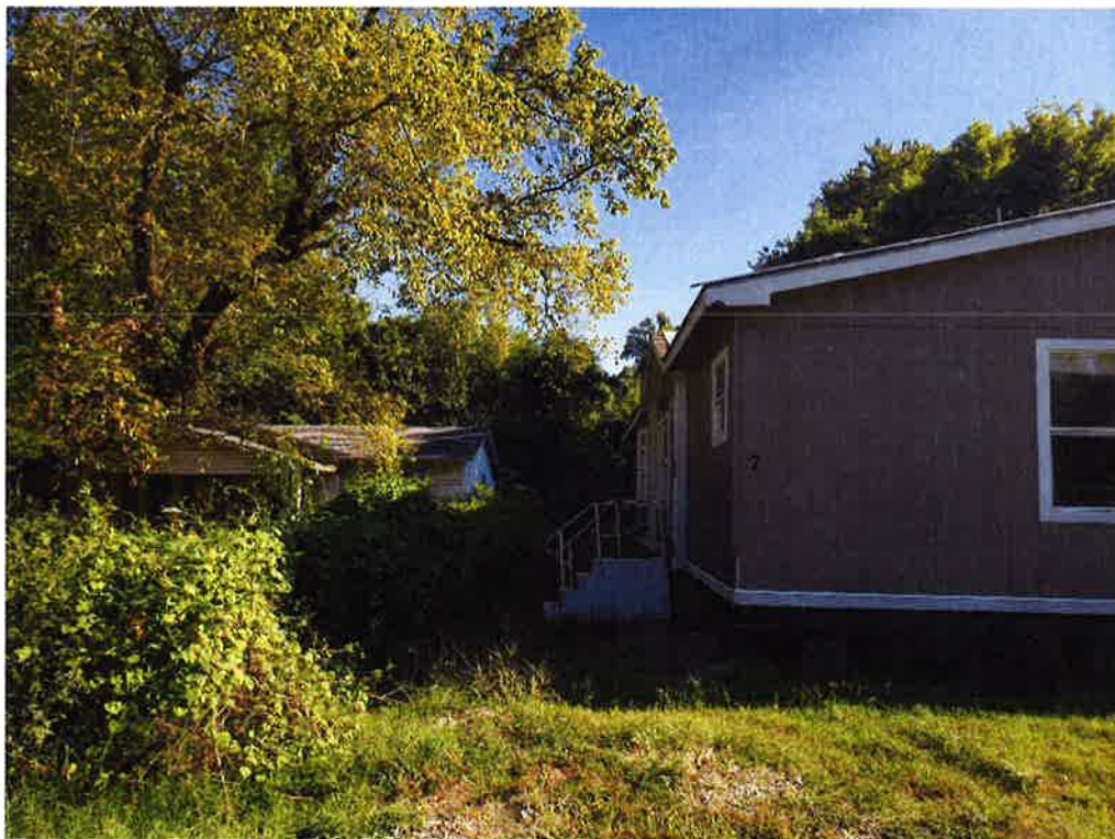
Looking south from W. 4th St. N.
