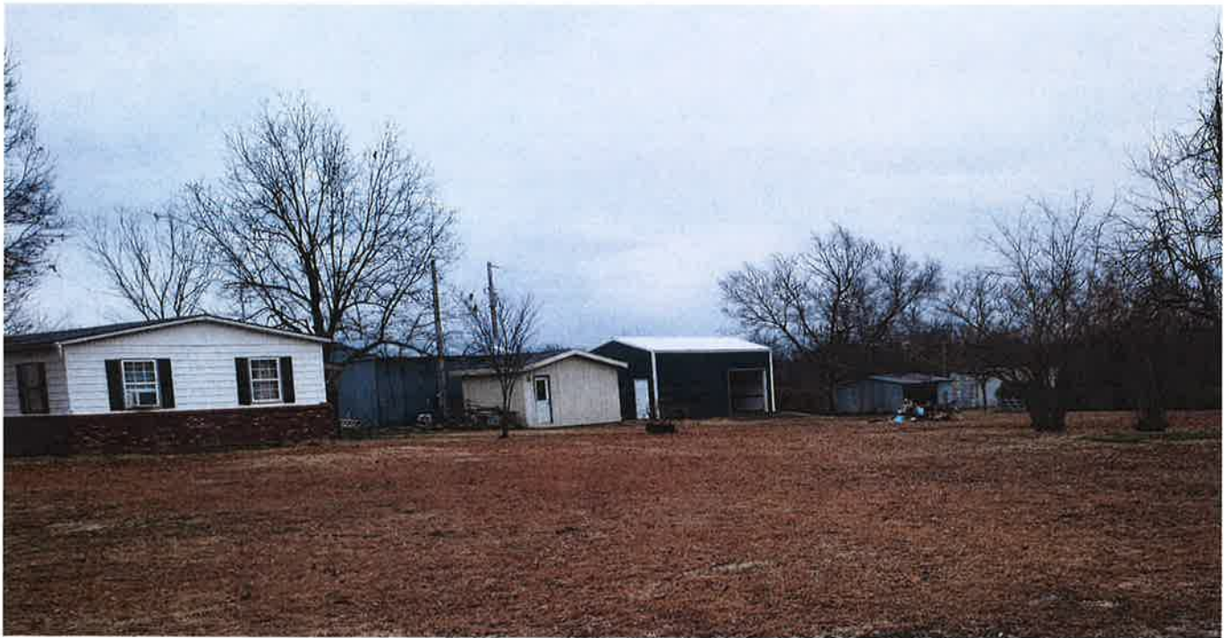
Looking northeast from N. 143 rd E. Ave. toward location of the existing and proposed shops
