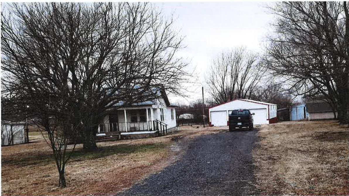
Looking west from N. 92nd E. Ave. toward site of proposed Horticulture Nursery
