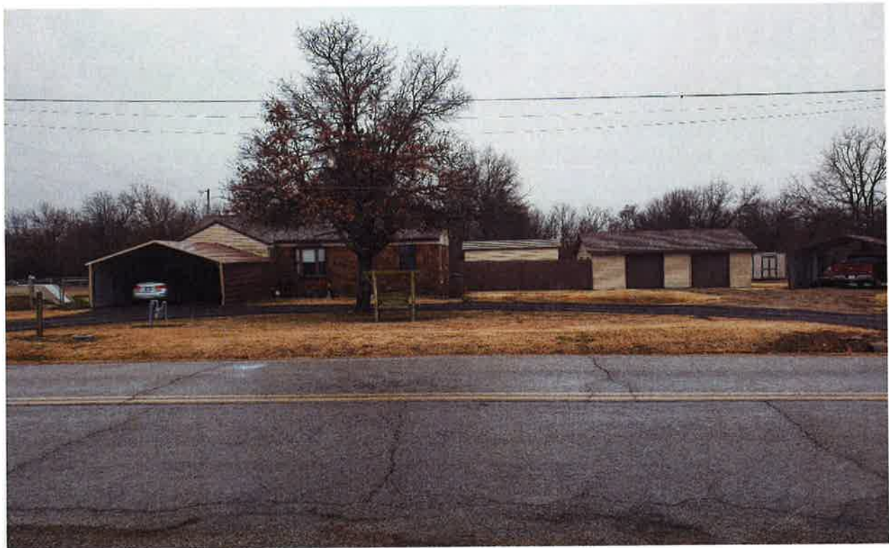
Looking south from West 41 st Street South at subject property
