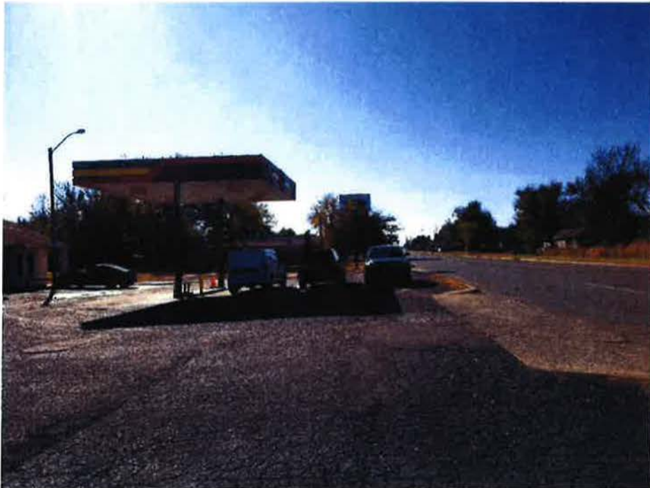
Looking south, the building is on the left.
