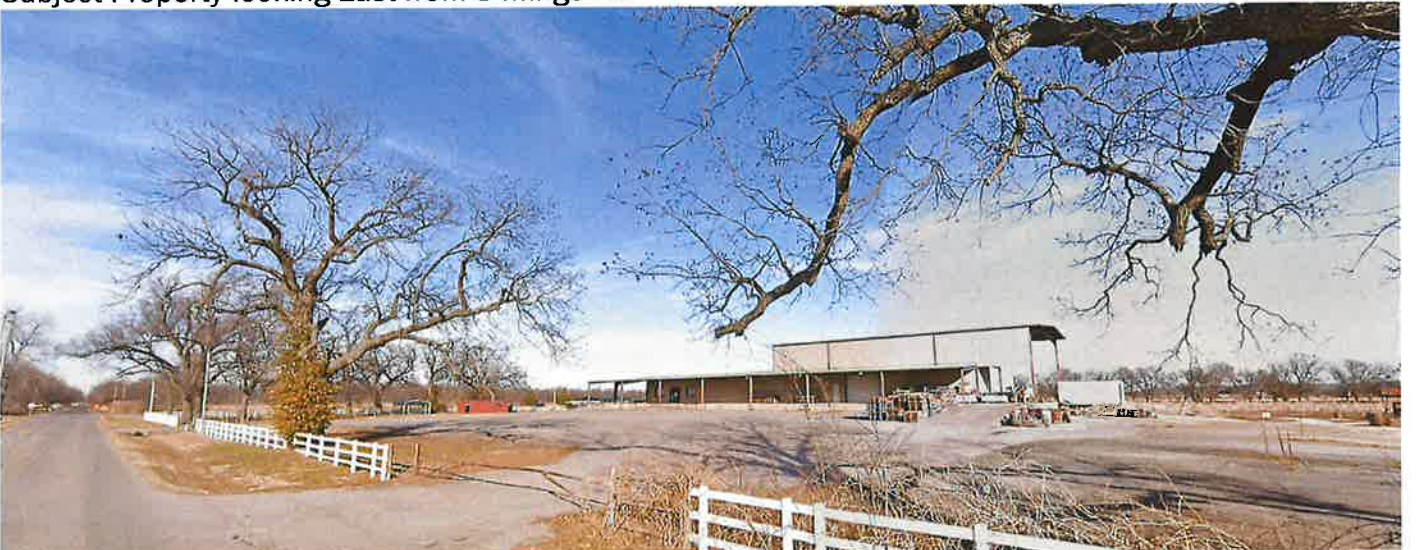
Subject Property looking Northeast from S Mingo Rd
