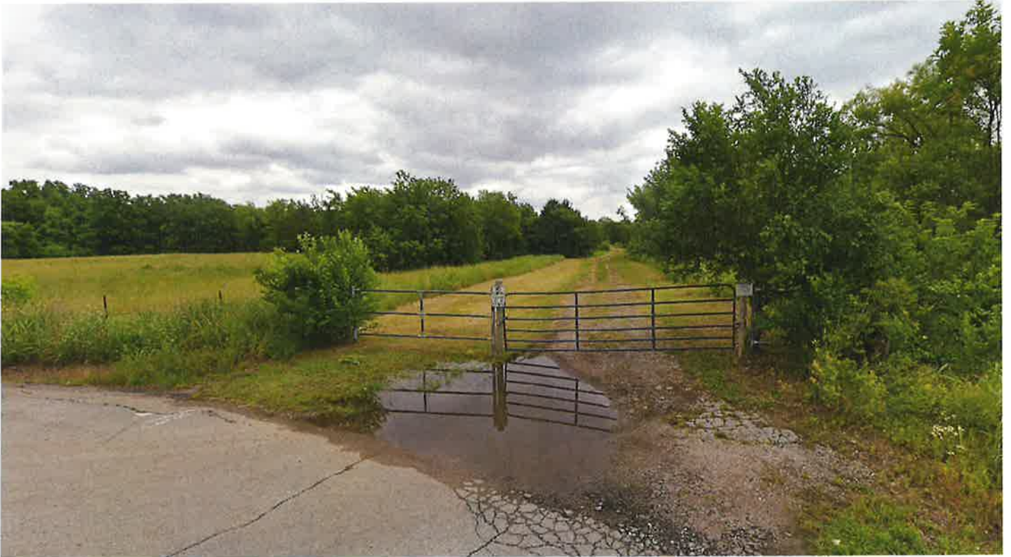
View of current access to subject lot looking East from S 45 th W Ave
