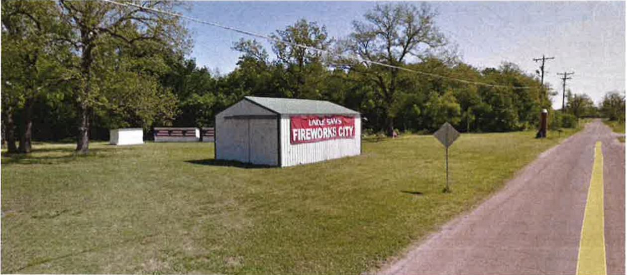
Looking northeast from E. 161st St. S. – image from Google Earth 2012
