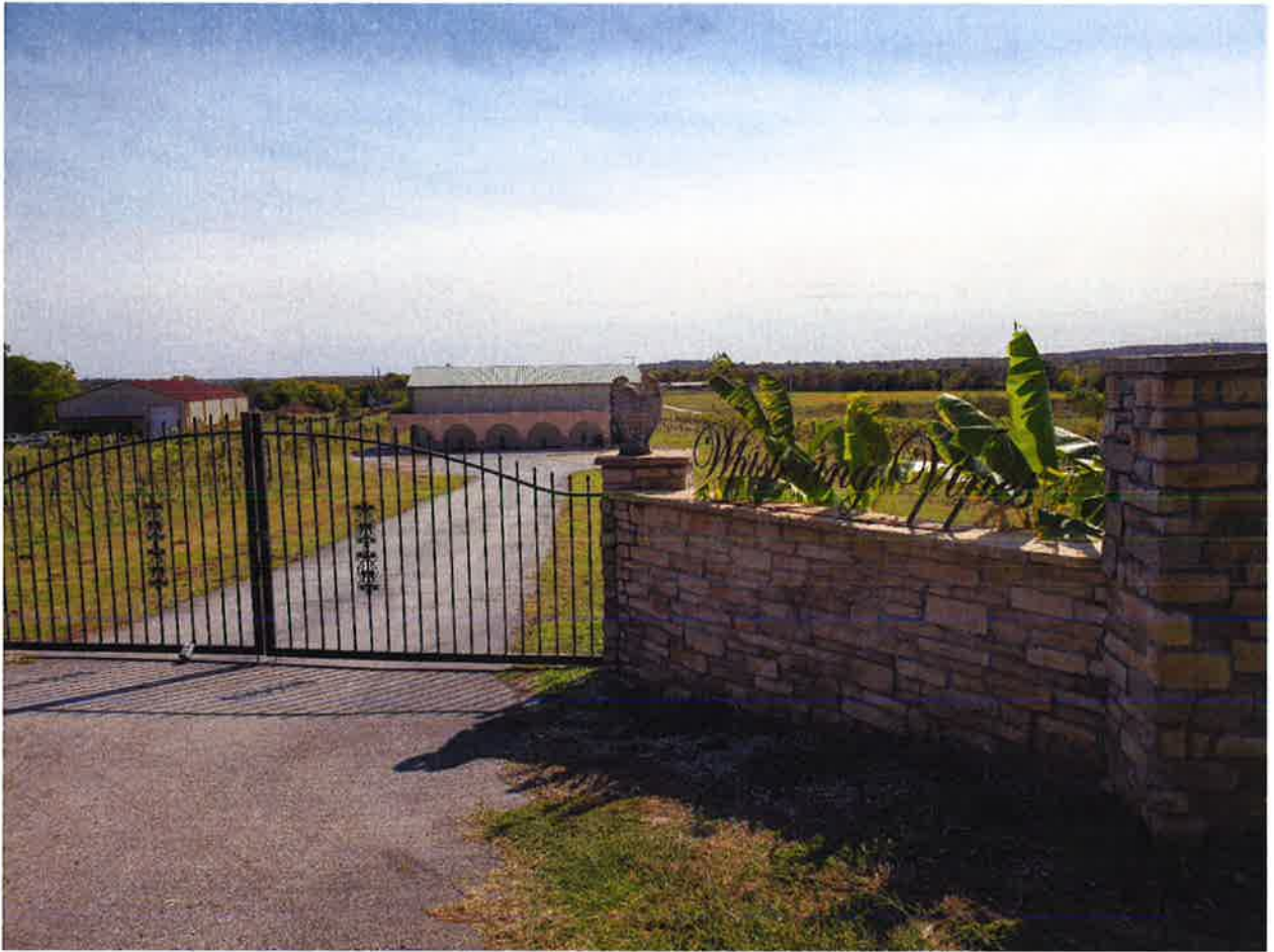
Looking south into subject property from W. 51st St. S.
