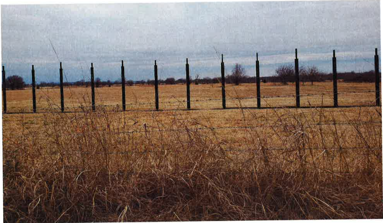
Looking west toward subject property from North Sheridan Road where the fence installation began in the front yard
