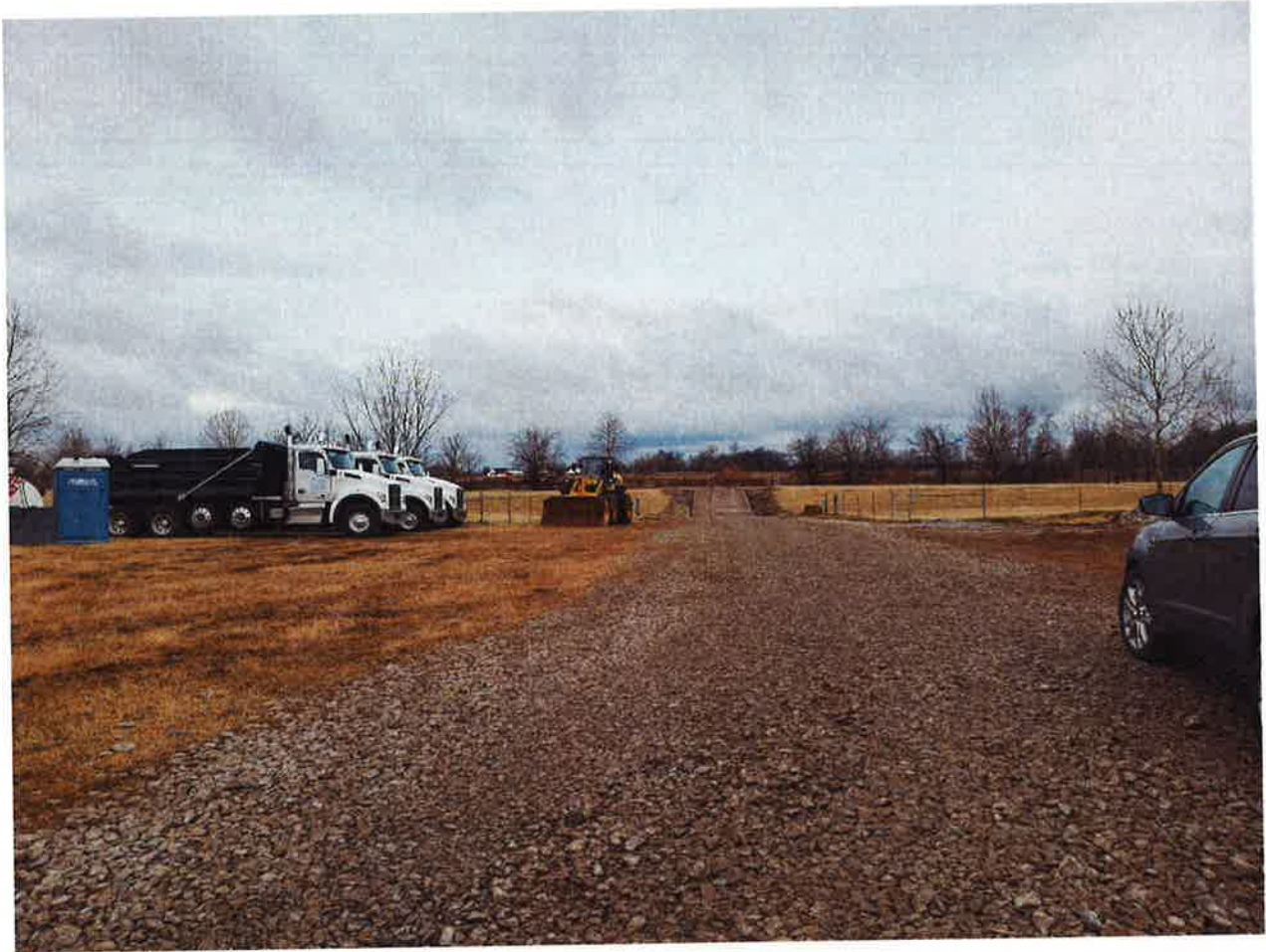
Looking north into entrance from East 161 st Street South
