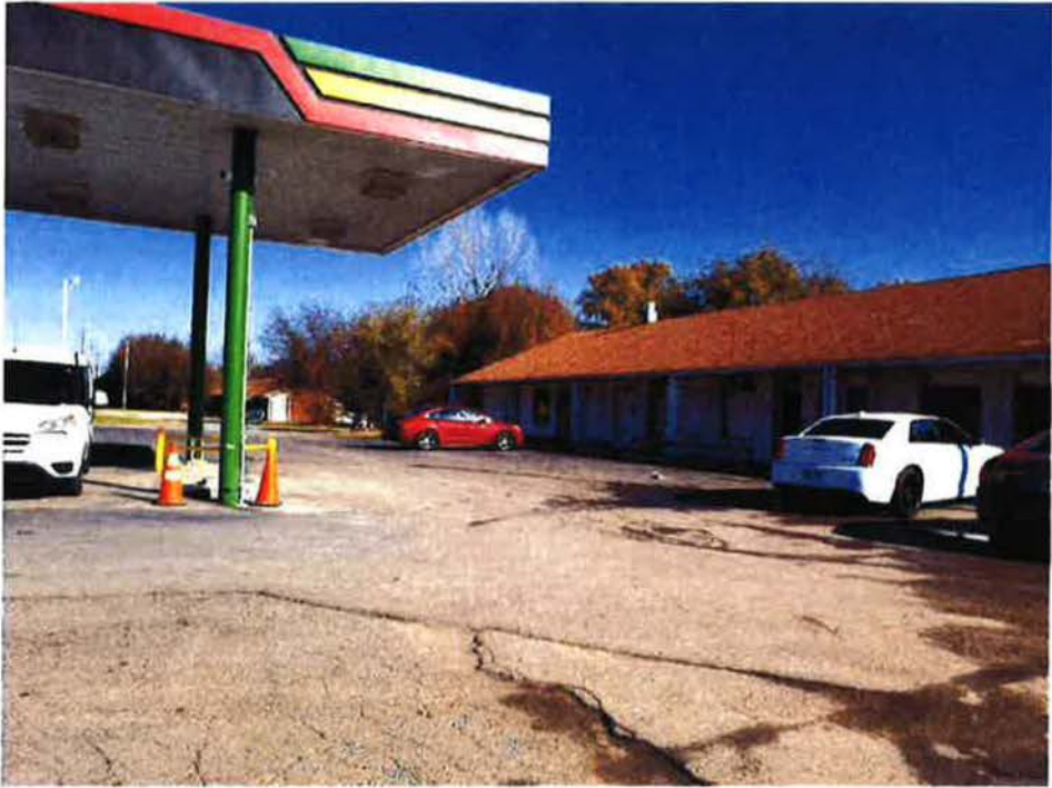
Looking north, the building is on the right.
