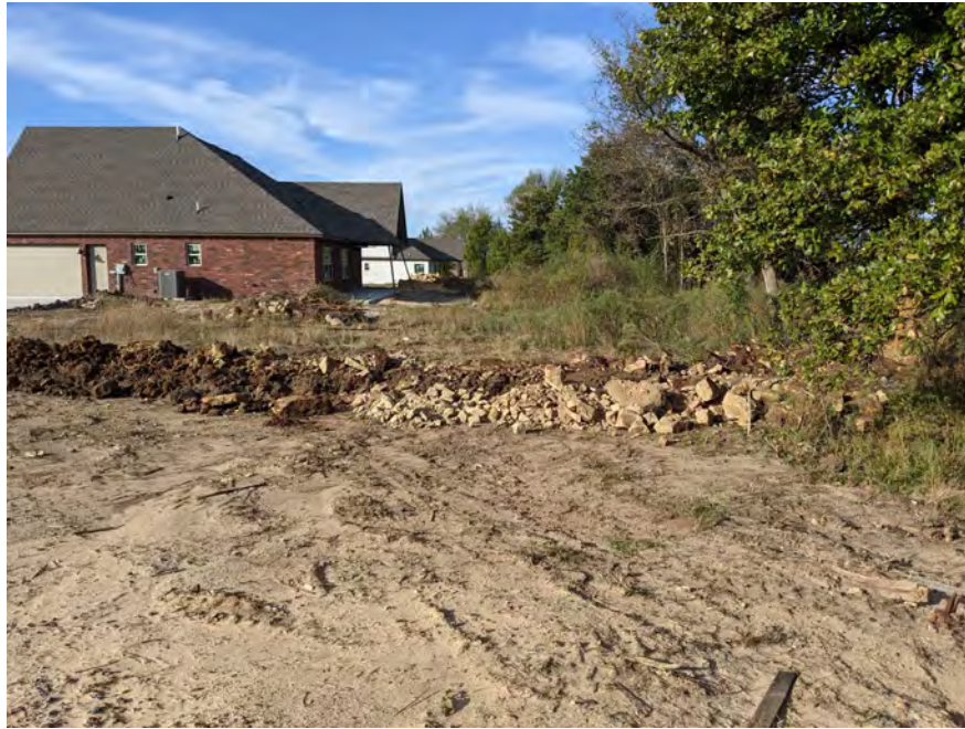
View behind house looking North during waterline relocation
