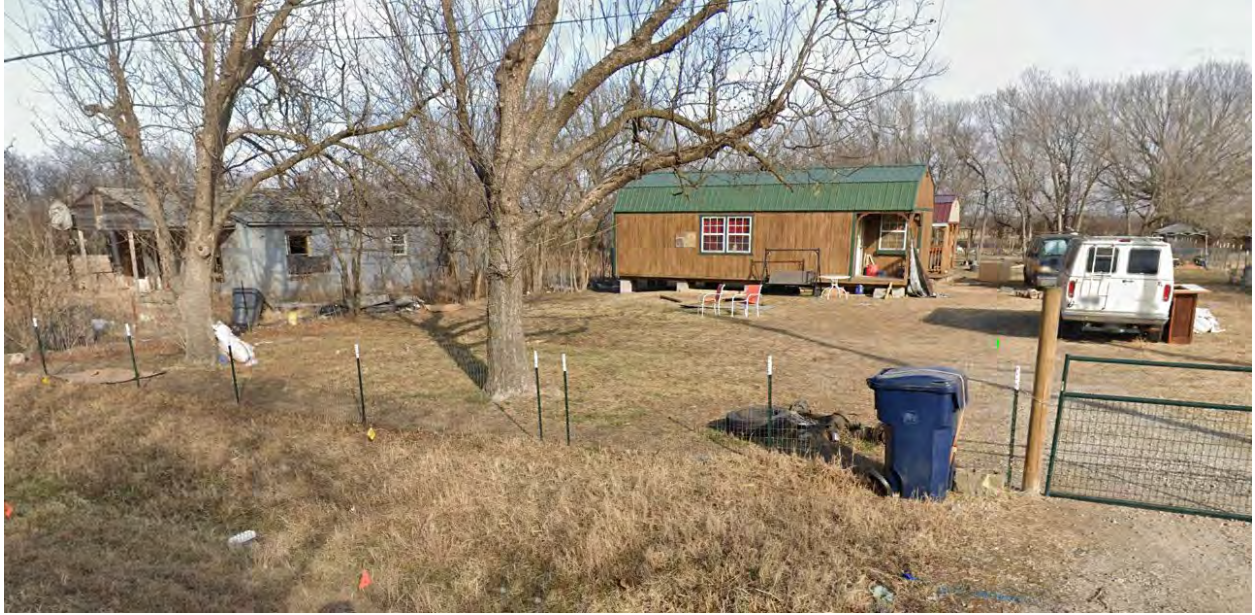
Looking east toward subject property
