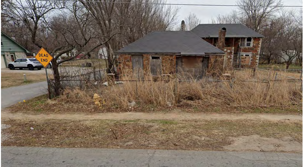
Looking east toward both dwelling units from S. 65th W. Ave.
