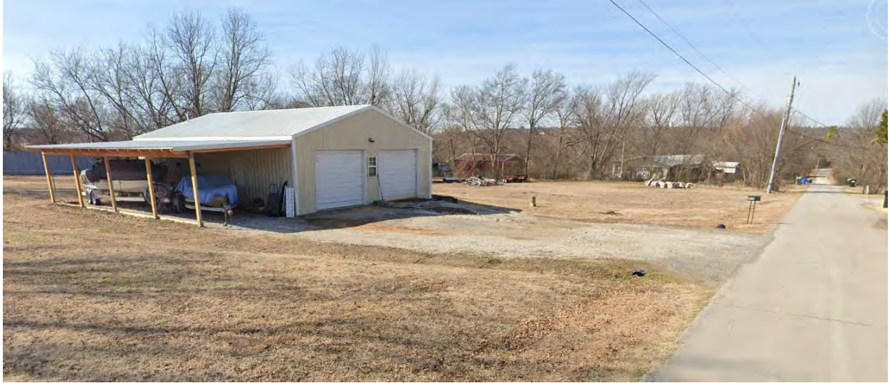
Looking west on W. 114th St. S. at the metal shop on the subject tract. The proposed additional dwelling unit would be just west on this structure.
