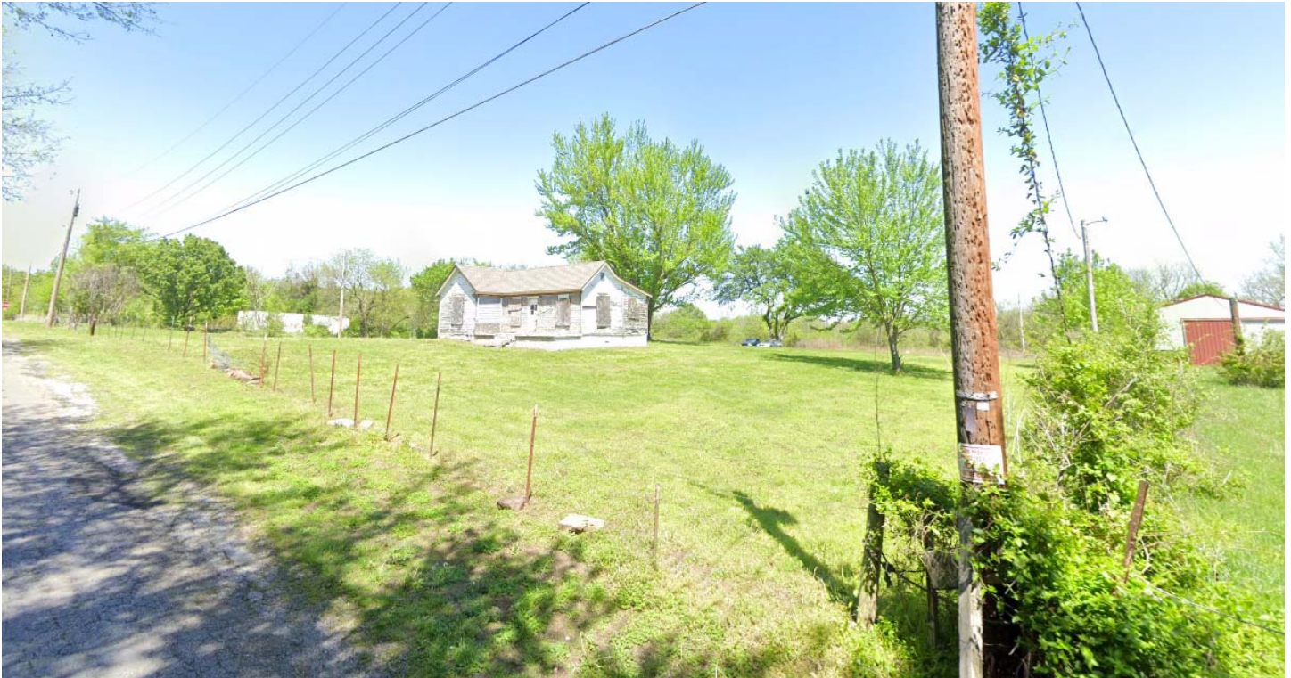
Subject Property looking Northeast from N Garrison Ave
