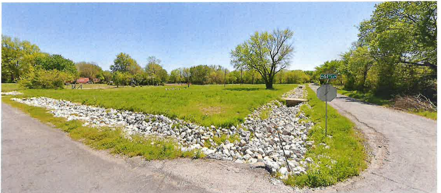
Subject tract looking Southeast from E 61 st St N
